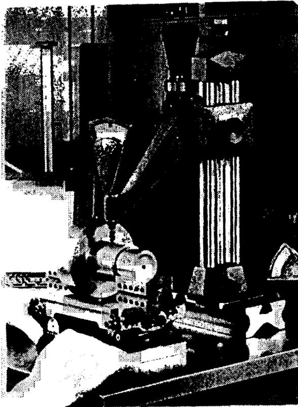
Fig. 79. Checking a Taper with Comparator and Sine Plate
